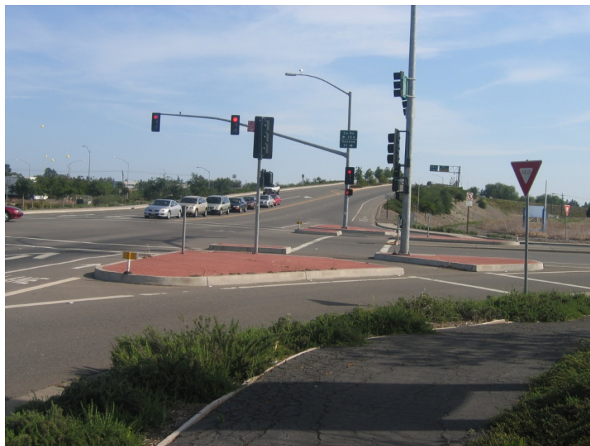
FIGURE 6 - Safe Intersection for Right Turns on Red
