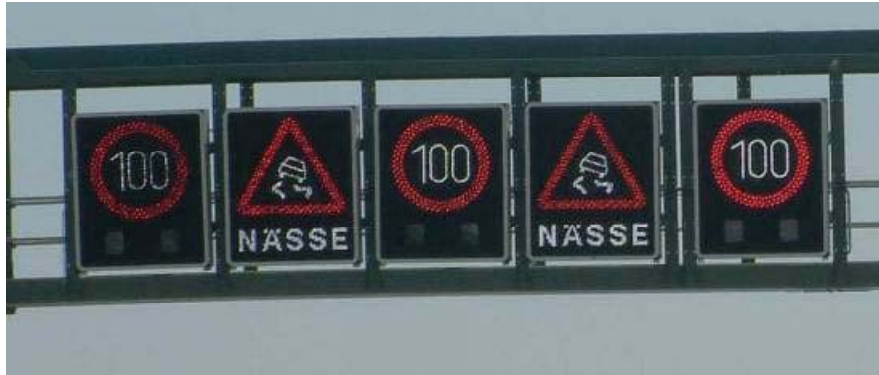
FIGURE 2a - Variable Speed Limit Gantry - Source: Boice et. al., 2006
